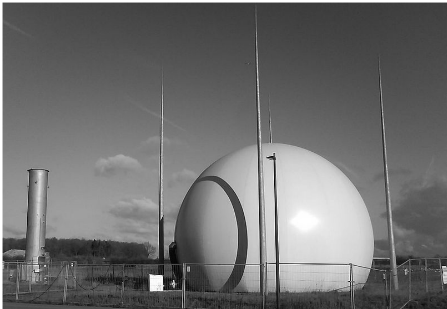
Figure 5.36 Pressurized gas storage tank.
