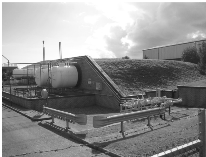
Figure 5.34. Mounded underground tank, courtesy BNH Gas Tanks.
