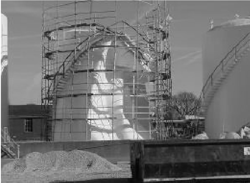
Figure 5.32. Tank collapsed by vacuum.
