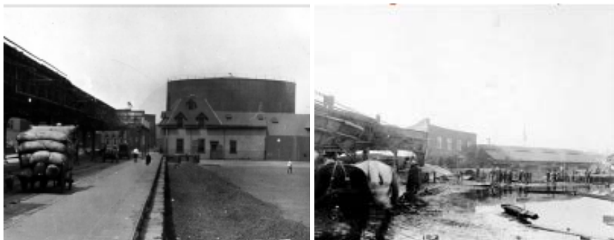
Figure 5.29. Molasses tank failure; before and after.
