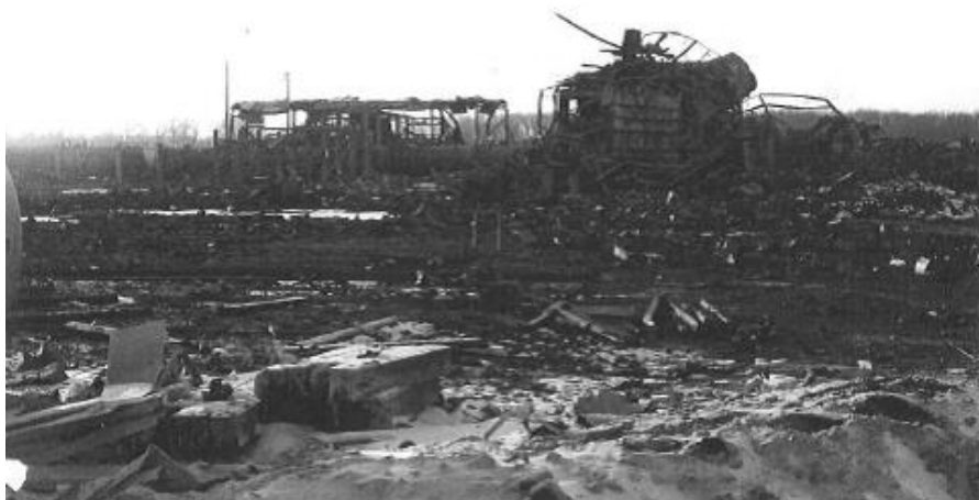
Figure 3.13. AN plant area after explosion, source, (EPA 1996).
