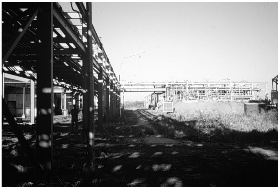
Figure 3.37. Photograph taken shortly after the incident. A pipe rack is shown on the left and the partially buried storage tanks (three total) for MIC are located in the center of the photo right, (source Willey 2006).
