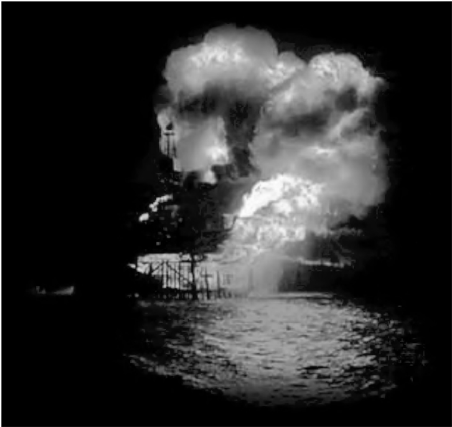
Figure 3.14. Piper Alpha platform, source (CCPS, 2008).
