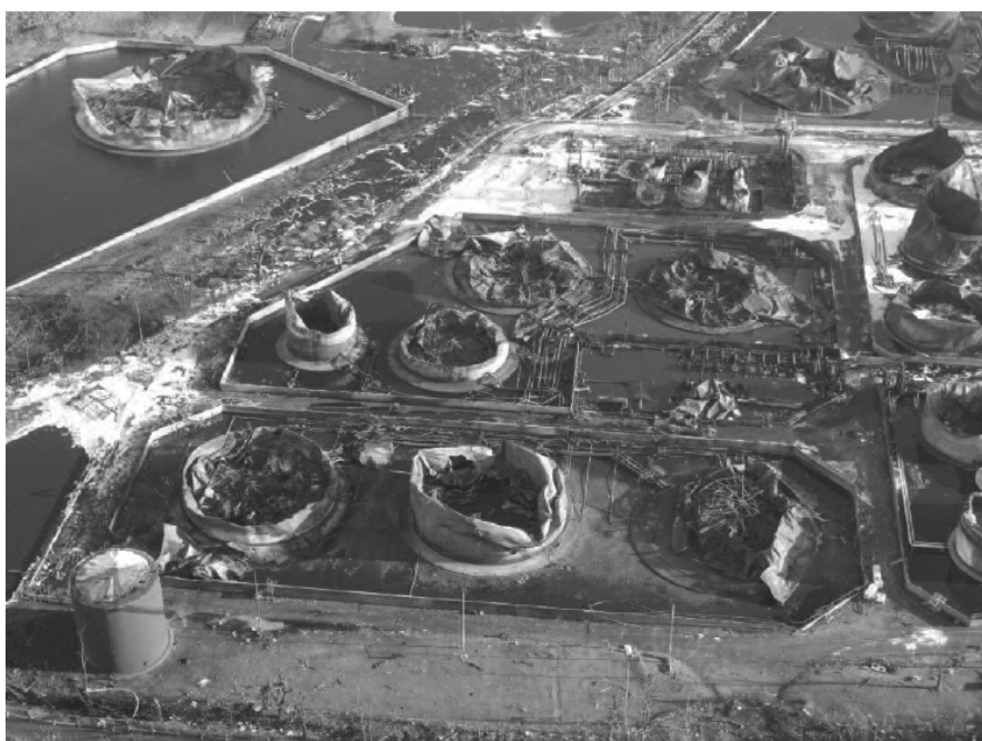
Figure 5.28. Buncefield after the explosion and fires, Ref 5.32.
