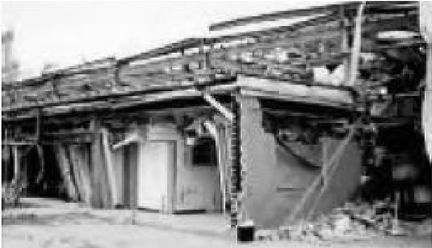
Figure 3.26. Damage to Flixborough control room.
