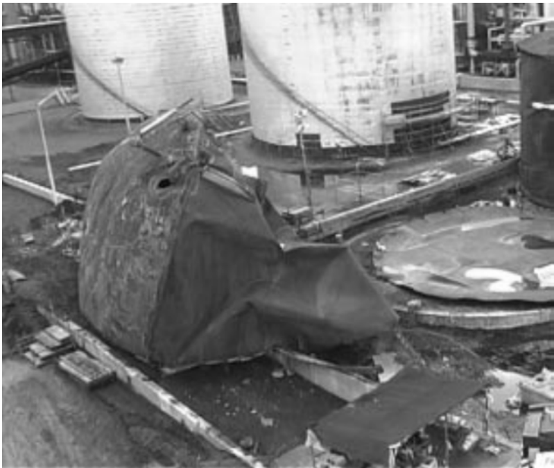
Figure 2.6. Collapsed tank at Motiva refinery, courtesy CSB.
